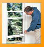
Note: Windsor's Revive sash replacement kits are designed to replace wood double hung windows. The wood side jamb pocket depth between the inside stop and the outside stop MUST measure at least 3-3/8" to accommodate the Revive sash replacement jambliner and clip.
